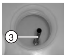
Overflow pipe on the fresh water tank
