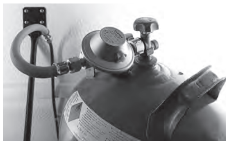
Connecting the gas regulator to the gas bottle
