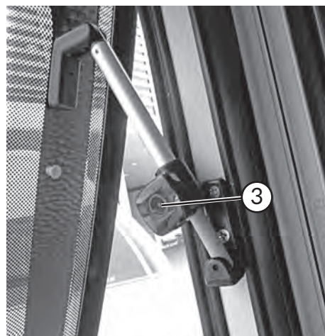
Fully adjustable window stays
