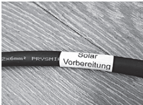
Preinstallation of the cable for the solar system
