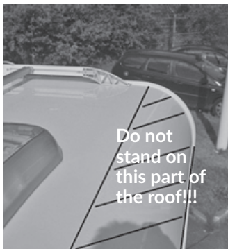
Curved edges of roof
