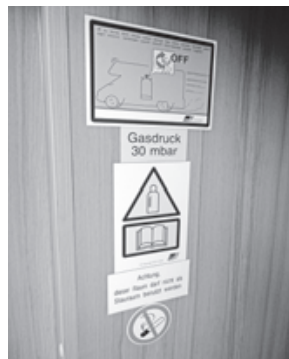
Safety instructions in gas bottle container
