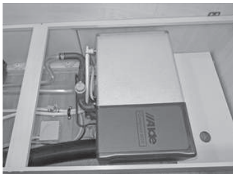
Alde hot water heating system
