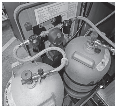
Extendable gas bottle container DuoControl CS
