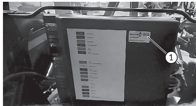
Central control panel with QR code
