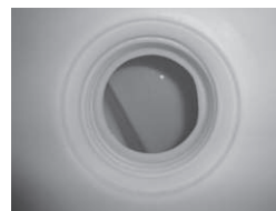
Fresh water tank
