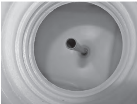
Overflow pipe of the fresh water tank
