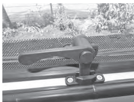
Window latch, in airing position
