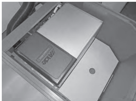
Alde hot water heating system
