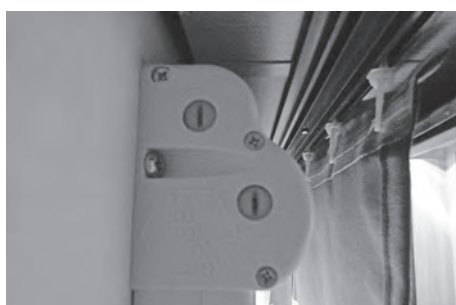
Retightening the tension spring on the shade
