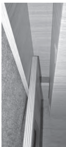
Wall panel on washroom wall
