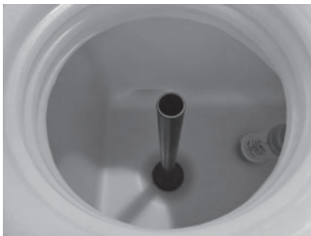
Overflow pipe of the fresh water tank
