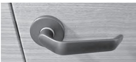
Washroom door handle
