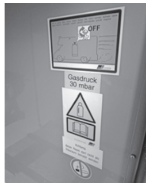
Safety instructions in gas bottle container
