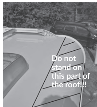
Curved edges of roof
