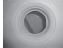
Fresh water tank
