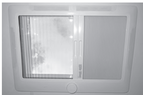
Large roof light
