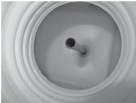
Overflow pipe of the fresh water tank
