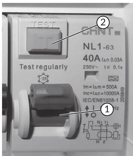
FI switch and test button
