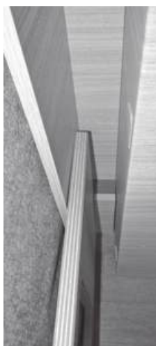
Wall panel on washroom wall
