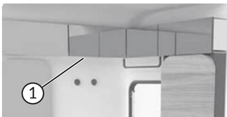
Wall cabinet in the washroom
