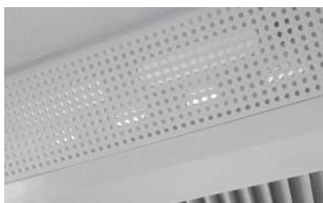
Forced ventilation of the roof bonnet
