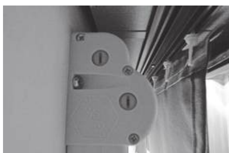
Retightening the tension spring on the shade
